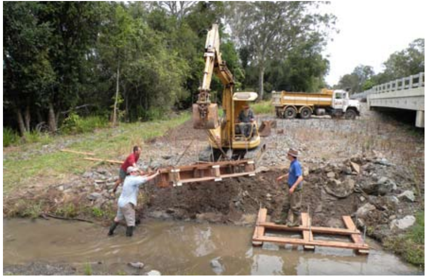
LUNKERs being lowered into position to provide stable aquatic habitat for fish and frogs in Belli Creek Crossing 2. [Photo by Eva Ford]
